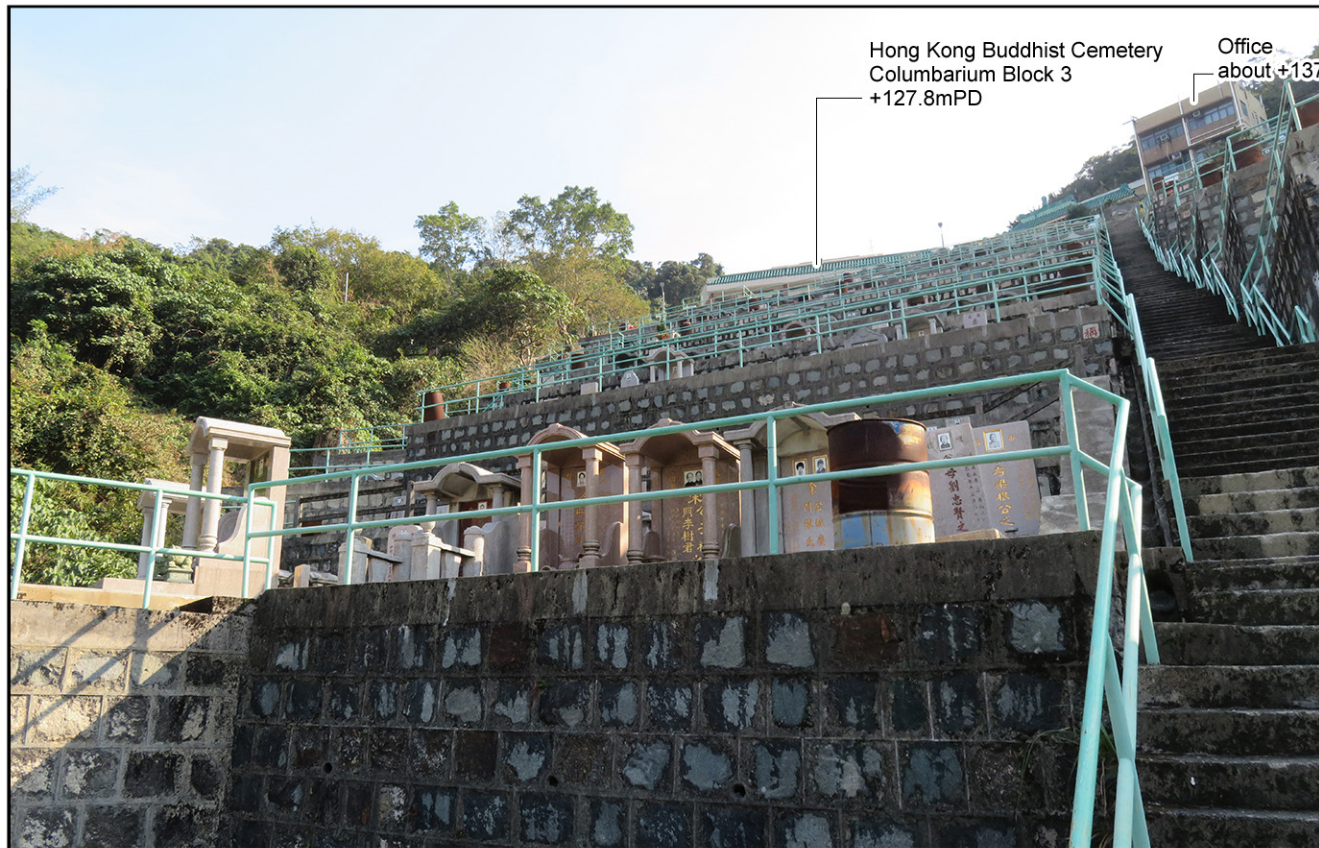
VIEW FOR EXISTING CONDITION
