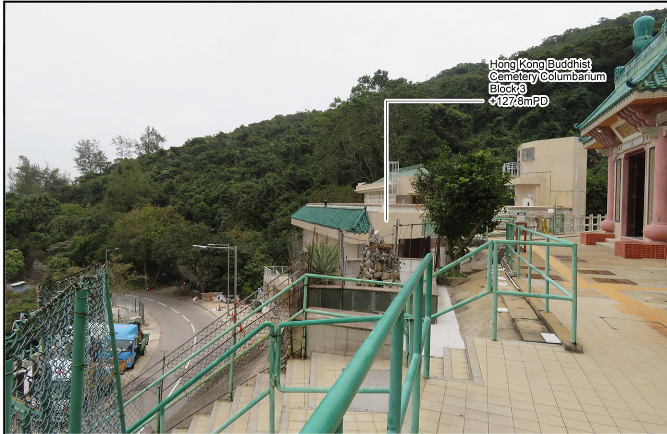
VIEW FOR EXISTING CONDITION
